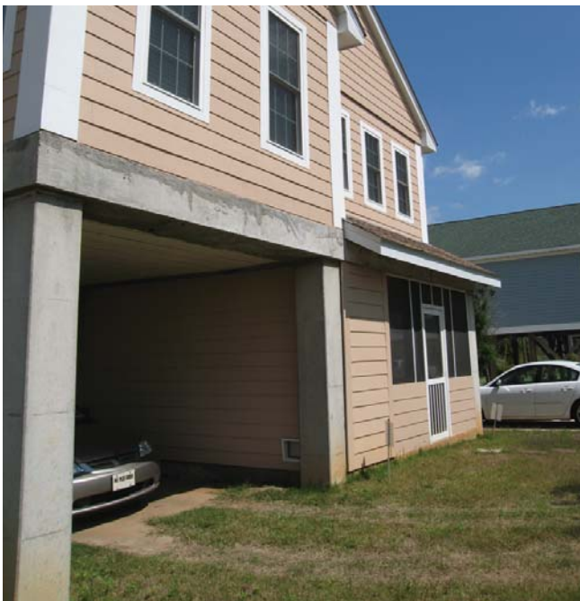
(Fig.14) This house is a good example of poured concrete piers using a square formwork, as opposed to round.
