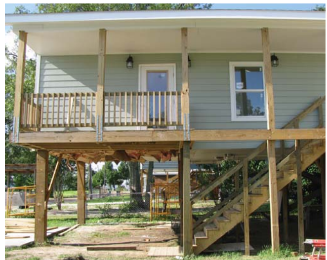
(Fig. 4) A house elevated on driven wood piles.
